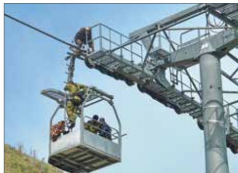
Cable car construction
