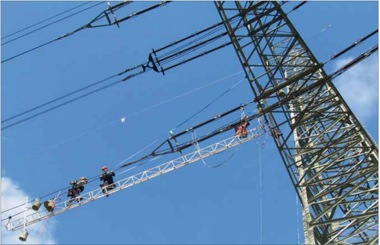
Overhead line construction
