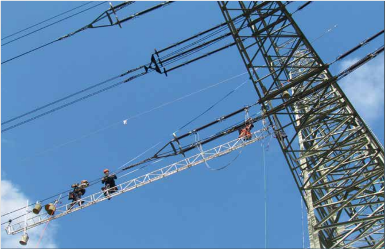
Overhead line construction
