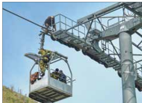
Cable car construction
